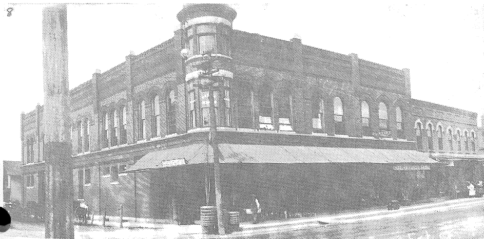
THIS EARLY DAY photo of the McNeill-Freese building in downtown Monticello was taken back in the days when the streets had a dirt surface. Note the hitching rails on the west side of the building. Eastwood Blvd. is now called Sycamore St. The building, housing McNeill's Hardware, Newhard's Clothing and Stuhler's Shoes, is located across from the Monticello Community building.
